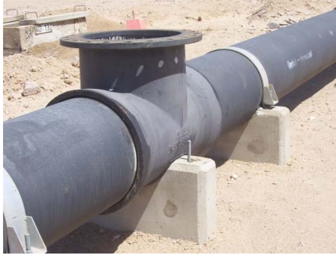
Figure 6: Provision made for an air valve on a 700 mm diameter water main
