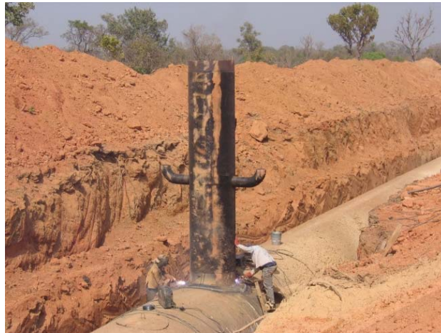
Figure 8: Installation in preparation for a staggered installation of air valves on a 3,5 m diameter pipeline
