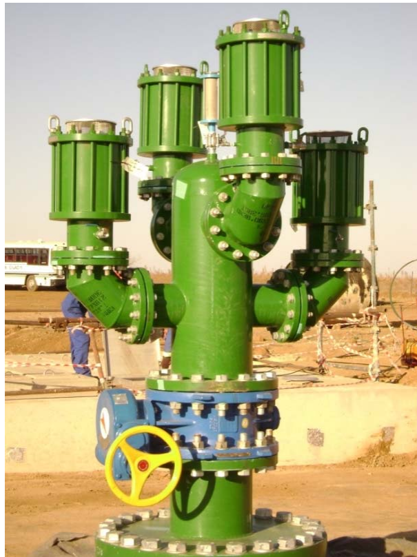
Figure 7: Staggered installation of air valves on a 1,9 m diameter pumping main
